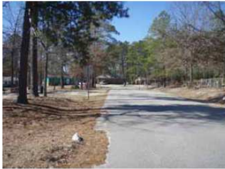
View Along Walter Hills Road (Photo Taken on February 14, 2012)
