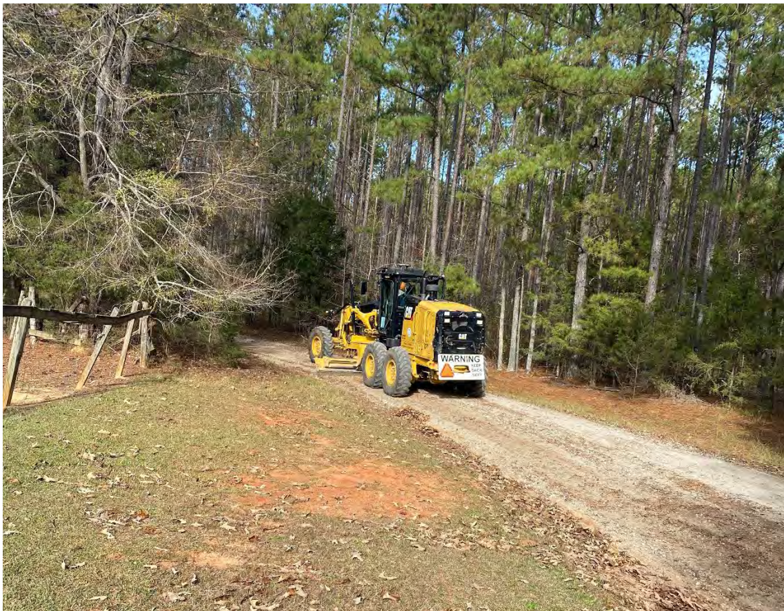
Unpaved road scrape performed by RDM crew
