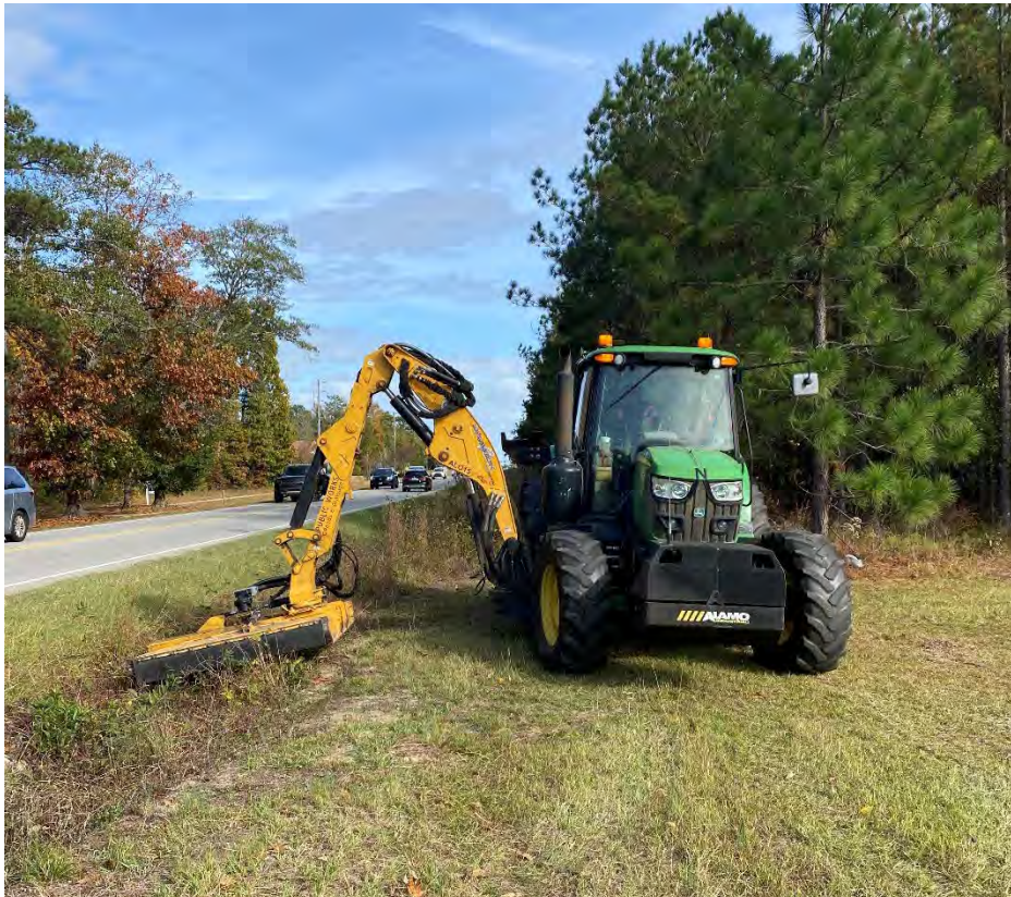
Slope mower cutting County right-of-way
