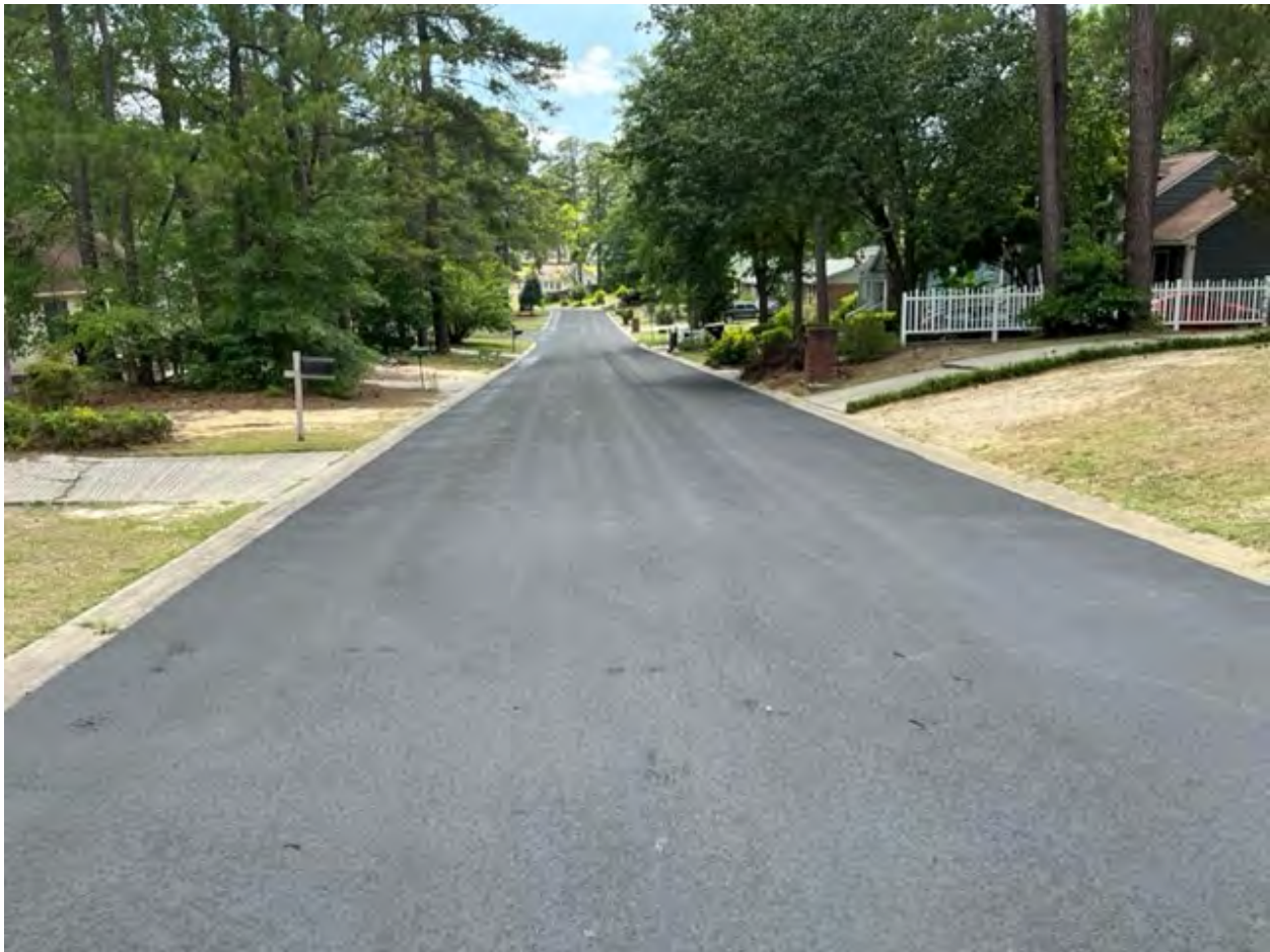
Pavement Preservation - New Castle
