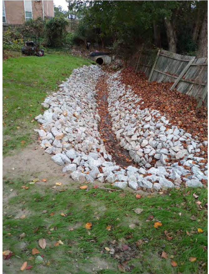
Morninglo ditch after maintenance
