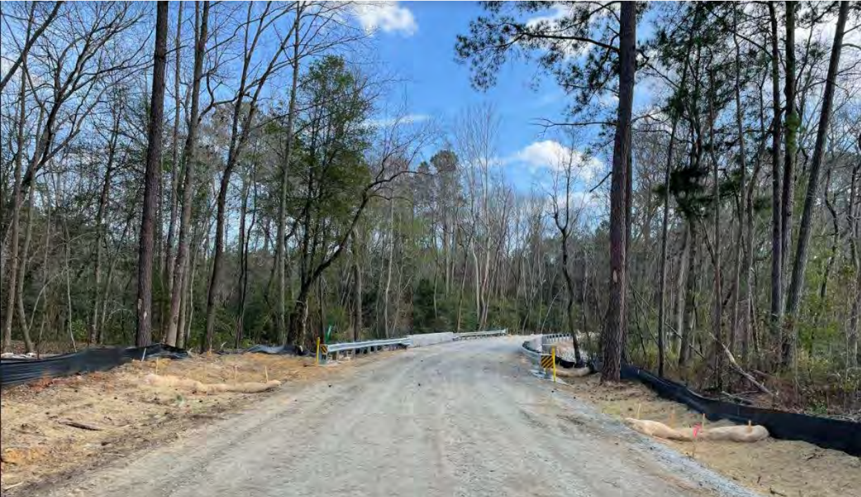
Countyline Trail bridge replacement
