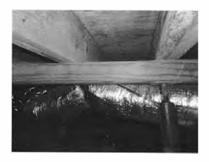
Picture 3: Shows the contractor able to observe past the duct work into the den upon removal of the floor joists in the kitchen and identify the issue with the floor joists in the den.
