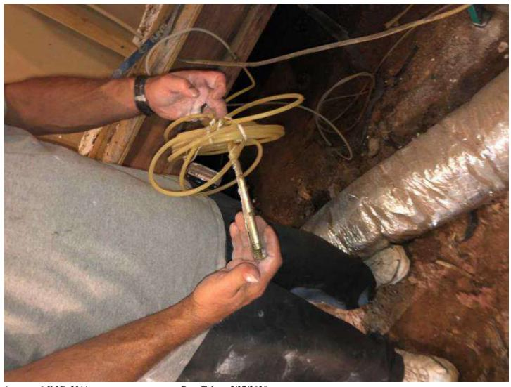
6 6-IMG\_3311 Date Taken: 5/27/2020 water line to refrigerator that was laying in the crawl space. disconnect ONLY and remove old leaking line.
